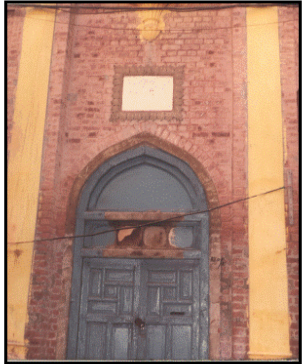
The ground floor portion of the building was donated to the Central Anjuman and it later also became the Central Library of the Anjuman.
